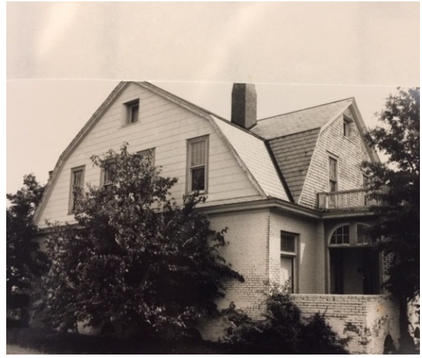
West Elevation Mayes House (1993)
