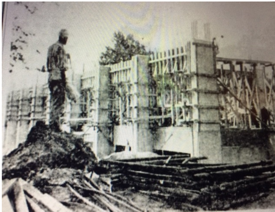
Central, Now Dowd Y.M.C.A, Under Construction (1959)
