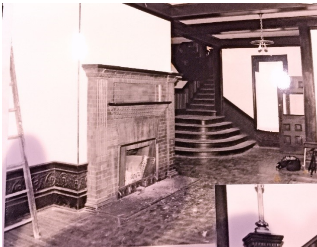
The Living Hall In Deteriorated Condition (1993)
