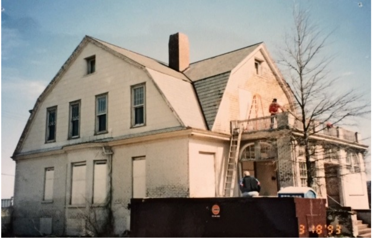
Workers Restoring The John And Idella Mayes House (March 18, 1993)
